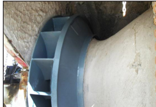
Installed fan coated with ARC
